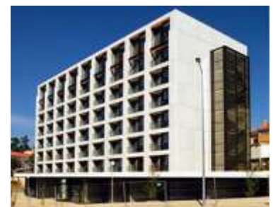
Studio Residence - Coimbra
